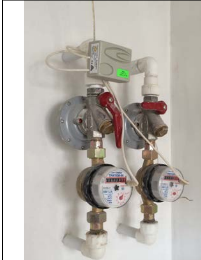
Water metering - two pulse inputs
